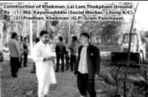
Construction of Khekman, Lai Lam Thokpham Ground By : (1) Md. Kayamuddin (Social Worker, Lilong A/C). (2) Pradhan, Khekman (G.P) Gram Panchayat.
